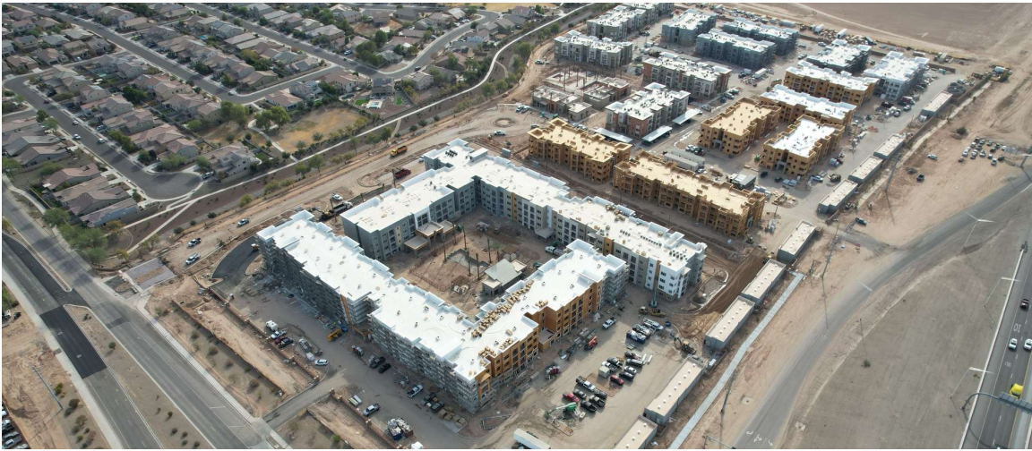
Estrella Springs and Suncrest Vista (Aerial photo 60% construction completion)
