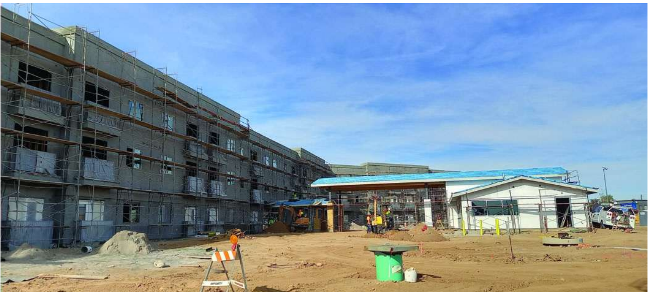
Heritage Senior Apartments (Overall view 40% construction completion)
