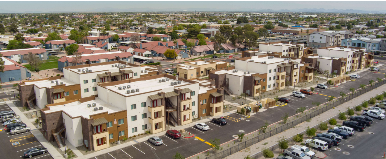
Norton Circle Apartments (Aerial photo post-construction)
