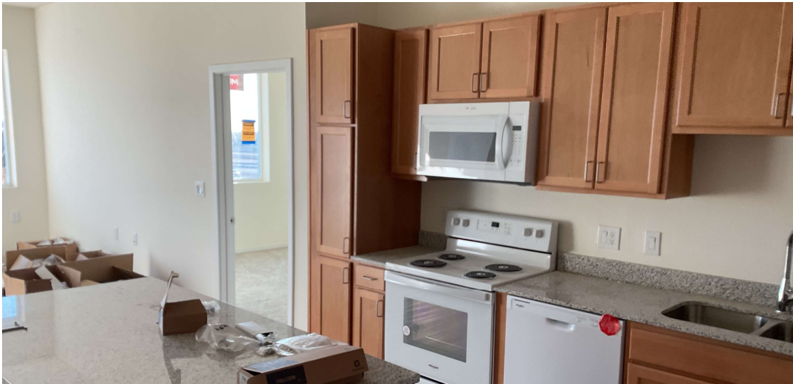
Suncrest Vista (Apartment interior photo 60% construction completion)
