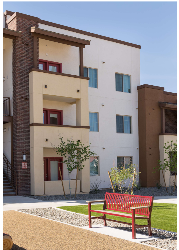
Inner Courtyard at Norton Circle Apartment
