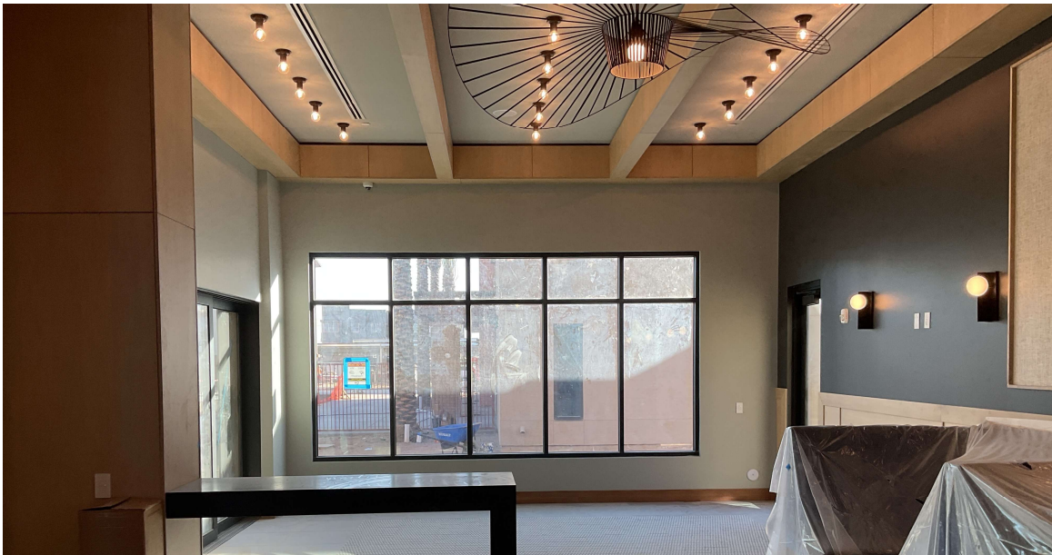
Estrella Springs (Community Space interior photo 60% construction completion)
