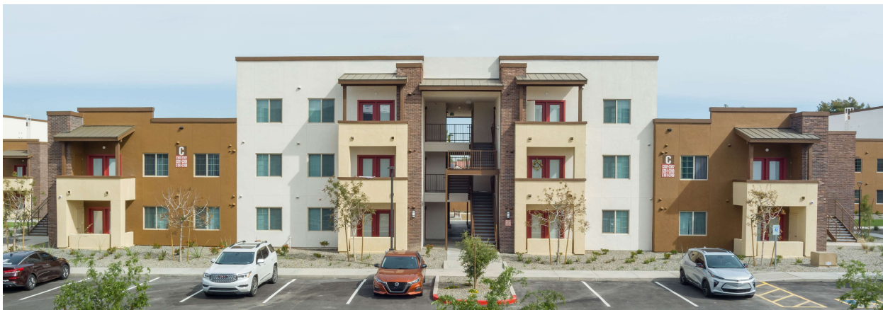
Construction Completion – Norton Circle Apartments Avondale, AZ
